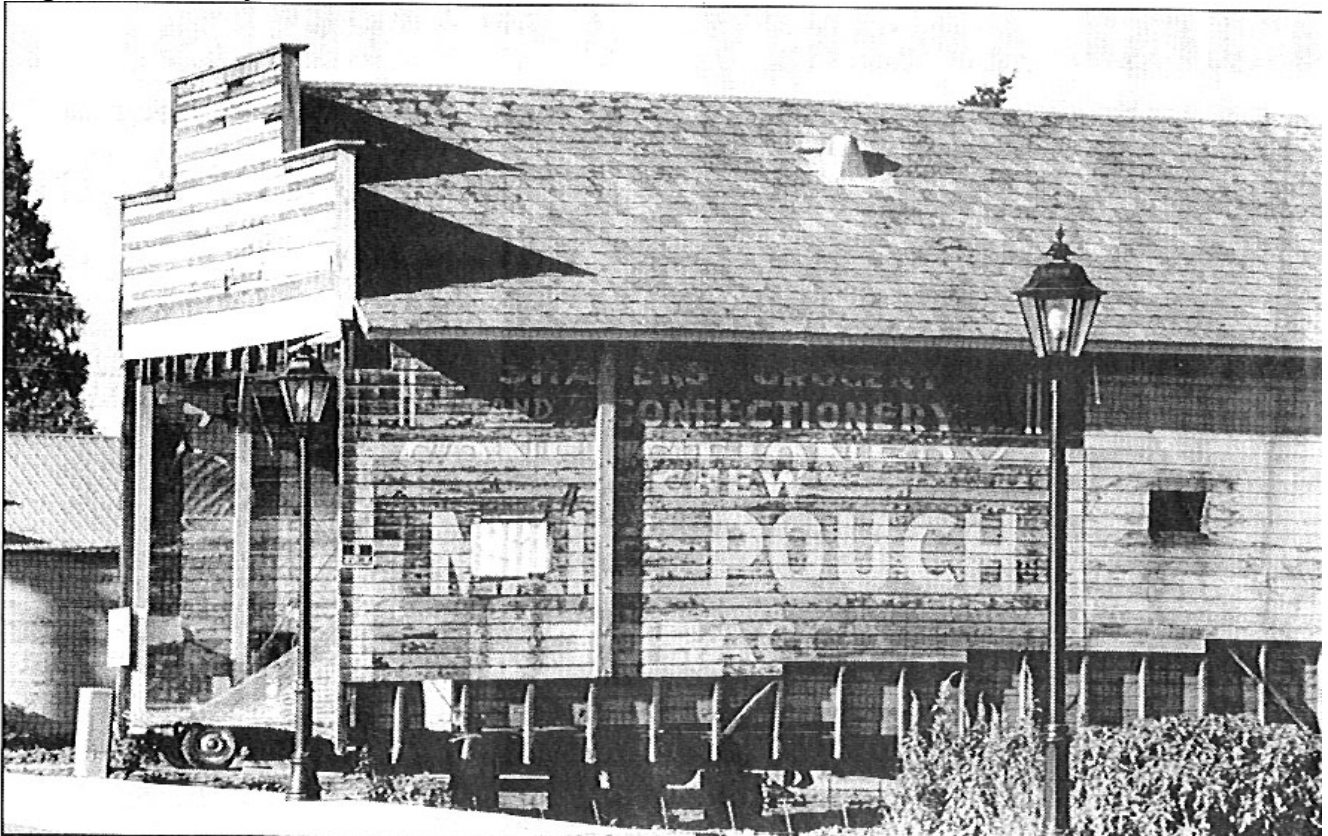
Hanscom Hall: former IOOF lodge on missing top floor, old Talent Cafe, post office, antique store, bakery, pottery studio, now Total Picture at 201 Talent Avenue. Built 1906
